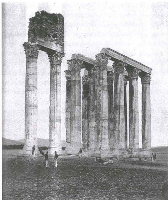
31 The temple of Zeus in Athens showing the remains of the medieval superstructure: Photographs by James Robertson: "Athens and Grecian Antiquities", 1853–1854, from the Photographic Archive of the Benaki Museum (© Benaki Museum, Athens, 1998) 113.
